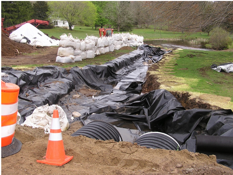
Culvert replacement on Ten Rod Road where it crosses the Queens River at the Exeter Country Club.
