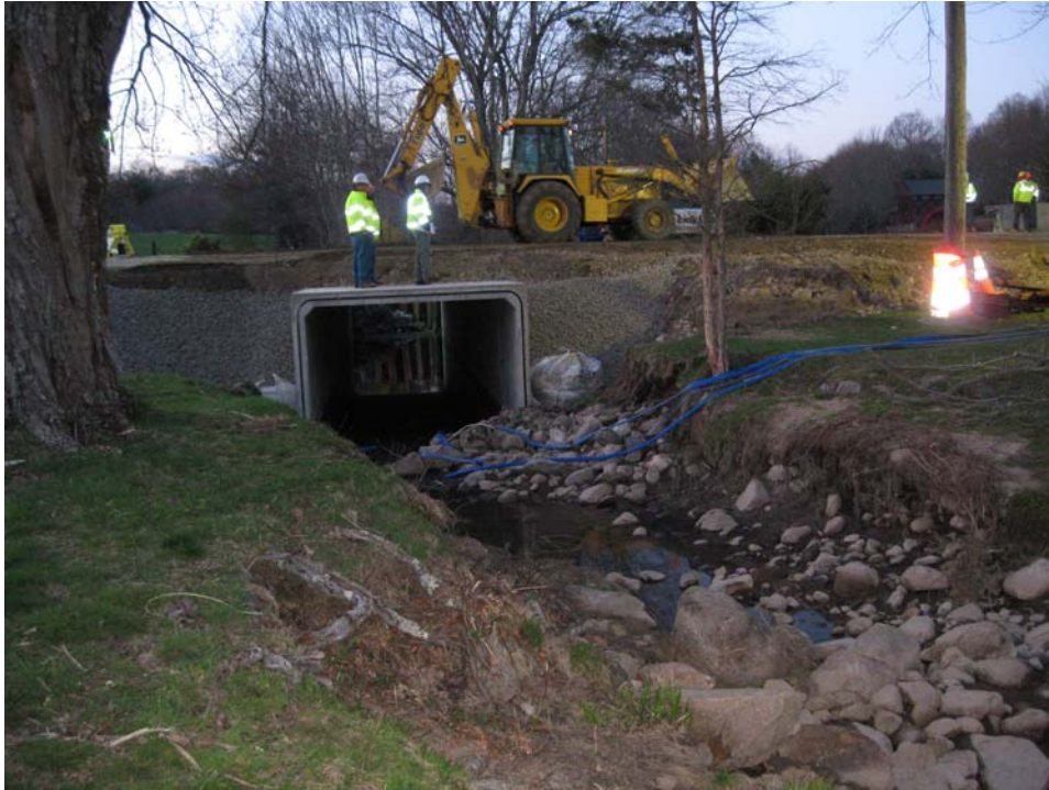
Culvert replacement on Ten Rod Road where it crosses the Queens River at the Exeter Country Club.
