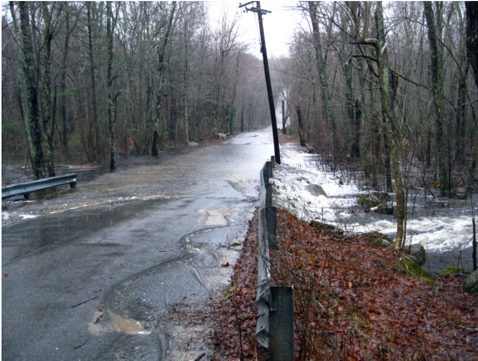
Parris Brook overflowing Old Voluntown Road. Photo courtesy of Sheila Reynolds-Boothroyd.
